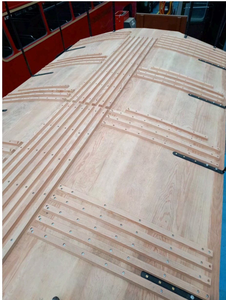
PHOTO CREDIT: ALAN GASKELL New upper deck floor
