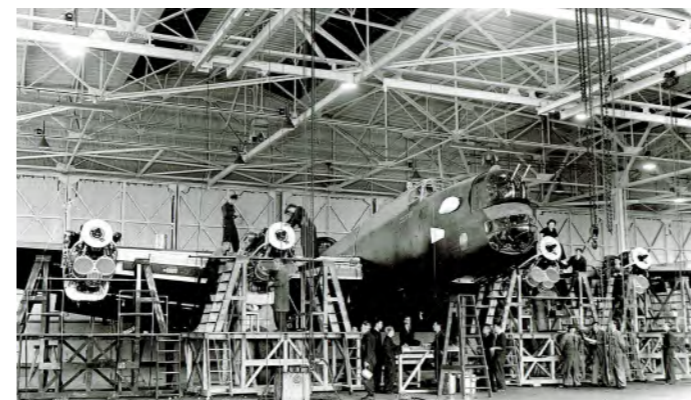
Final assembly of a Halifax underway in a Leavesden hangar
