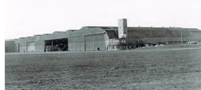
A general view of the main assembly hangars at Leavesden Airfield
