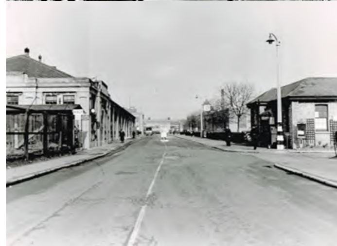
Chiswick Works during WW2
