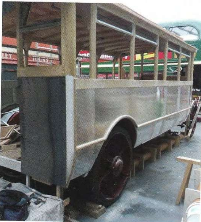
The lower deck panelling in place on NS174. (MHCB)
