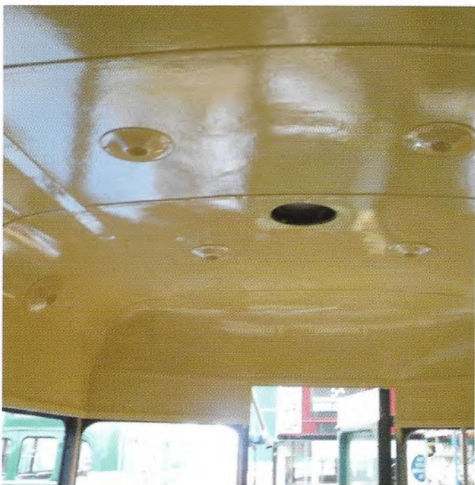
The ceiling now sporting its final topcoat.
