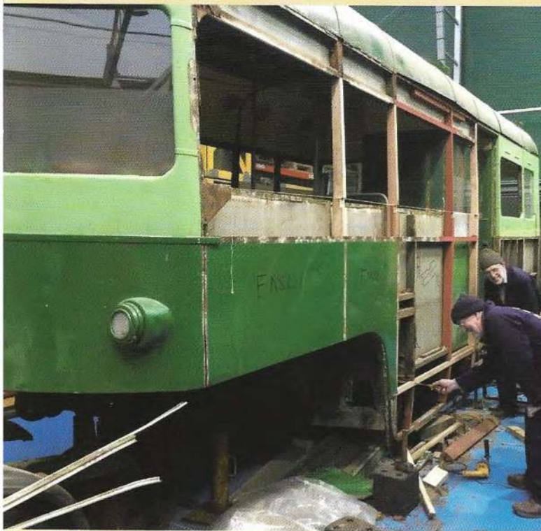
Above: Work proceeds in reframing the Canteen Trailer.
