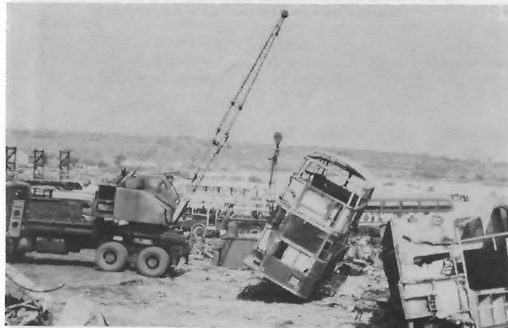
RT3096 later in the day receives attention from the crane
