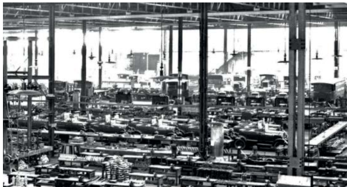
Inside the Leyland Ham Factory
