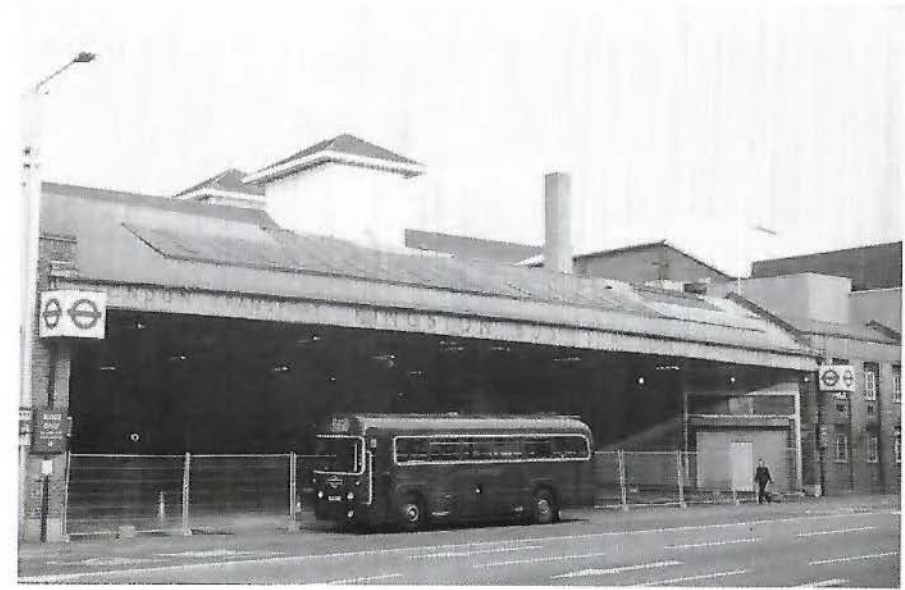
Top: It is anticipated that the LT Museum will rescue the 'General Omnibus Station' sign. Lower: RF672 pays its respects on behalf of all the enthusiasts that were drawn to the unique locale that was Kingston Bus Station Photos: CBM
